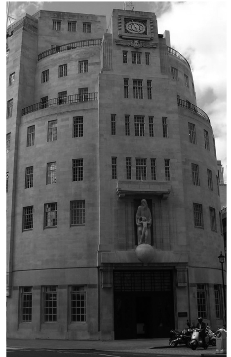
Broadcasting House: cuts will do harm
